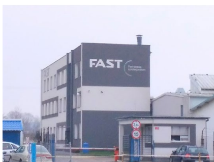
Current FAST plant.
